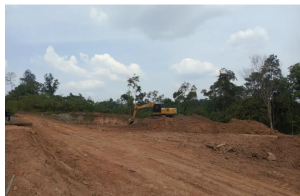
Initial site preparation and earthworks
