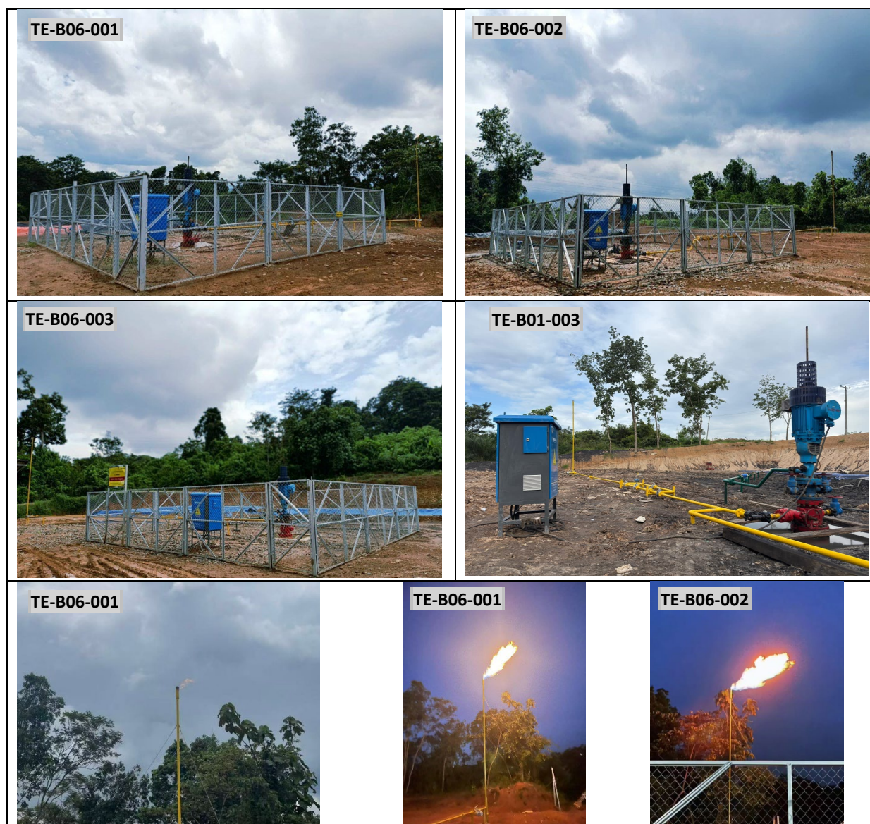
Dewatering and Gas Flaring Activities at Tanjung Enim Early Gas Sale
