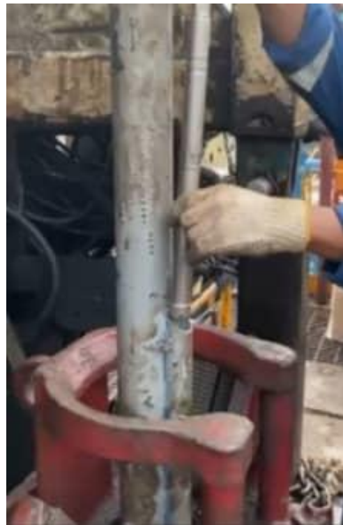
Completion Activity TE B01-003 installing PCP pump
