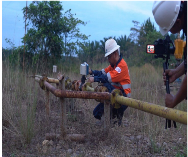
Regular monitoring to observe the gas rate readings and other relevant parameters during the dewatering process at MU-005TW
