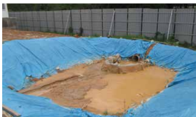
Silt Trap on Construction Site Reducing Water Pollution
