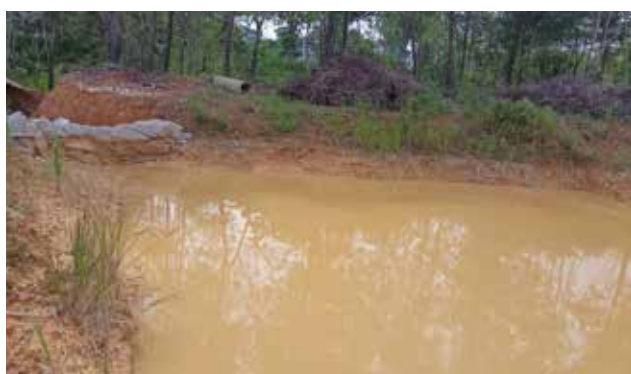
Silt Trap on Construction Site Reducing Water Pollution
