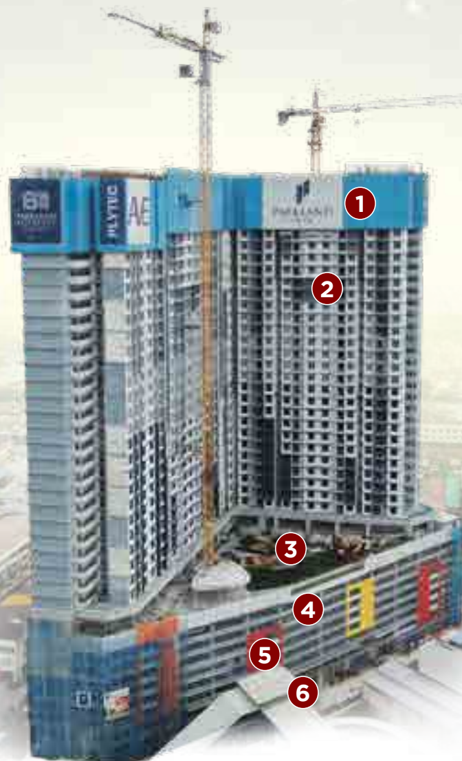
1 PLYTEC SCP (Self-Climbing Platform)
