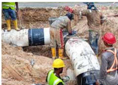
Trenching and installing water supply infrastructure piping
