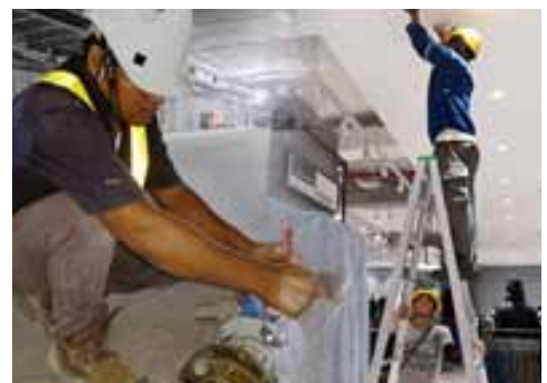
Personnel providing maintenance and repair services
