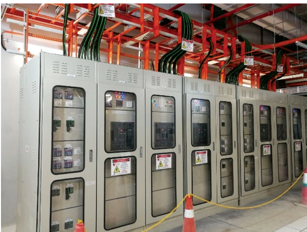
Power distribution system for a medical device manufacturing plant
