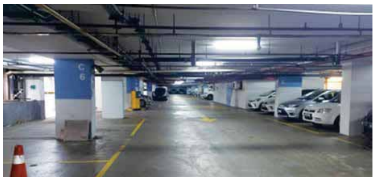
Figure 23-26: Plaza Mont' Kiara - Upgrade of basement car park lighting from fluorescent to LED lights.
