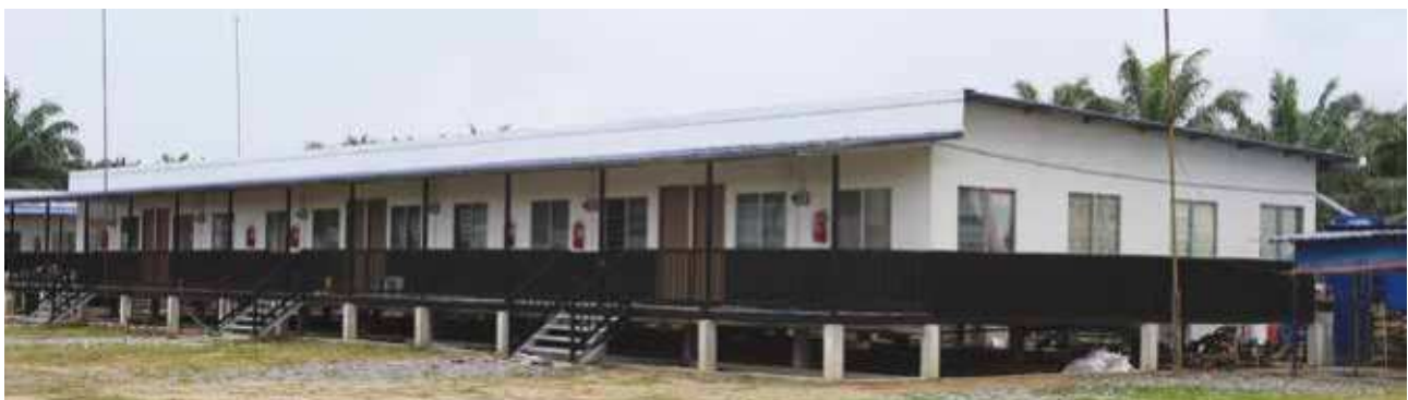
The Agro division's newly refurbished workers' quarters in Mukah, Sarawak.
