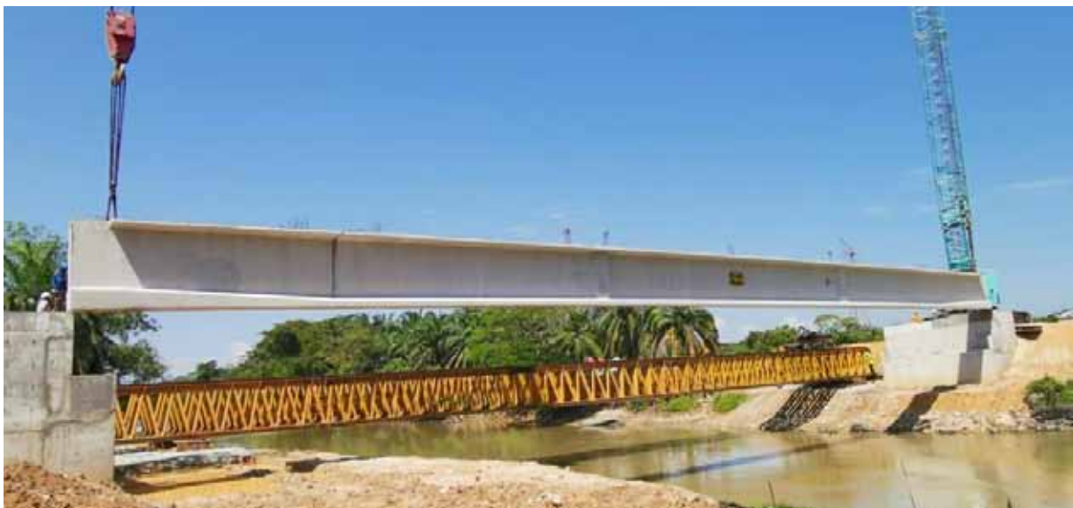
Picture: Launching of Long Span Girder at Jalan Air Kuning Tanjung Tualang, Perak Tengah to replace a wooden bridge
