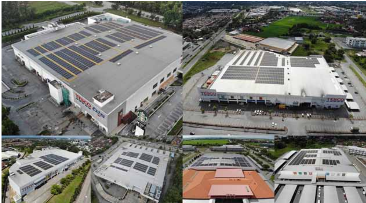
Picture: Solarvest has successfully delivered the largest hypermarket solar PV projects which include 15 designated Tesco (currently known as Lotus's) stores with a cumulative capacity of approximately 10,614kWp located across Peninsular Malaysia.
