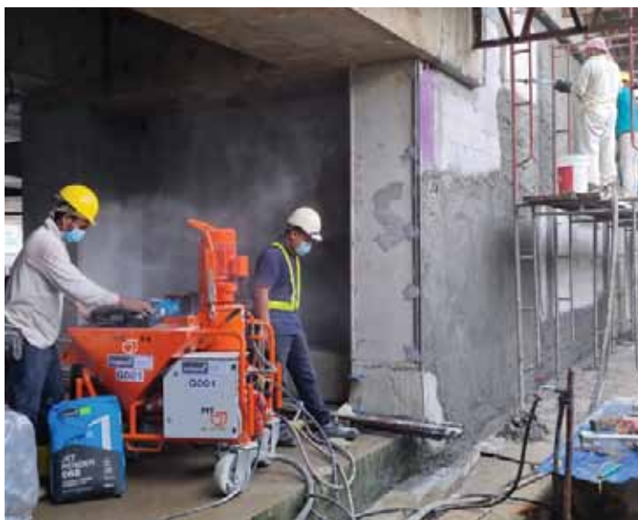
Picture: The application of spray Jet Render 668 at construction site.
