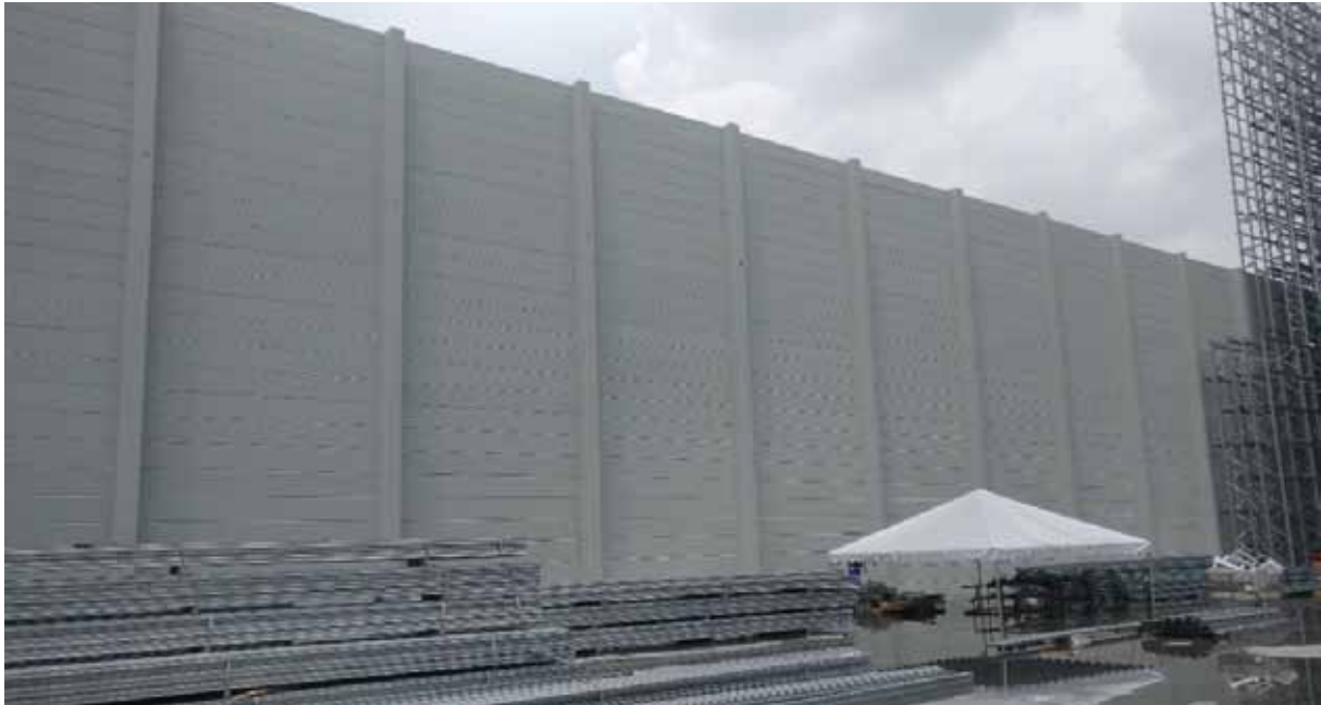
Picture: Starken AAC supplied the AAC panel wall as external wall to the Ikea, Klang.
