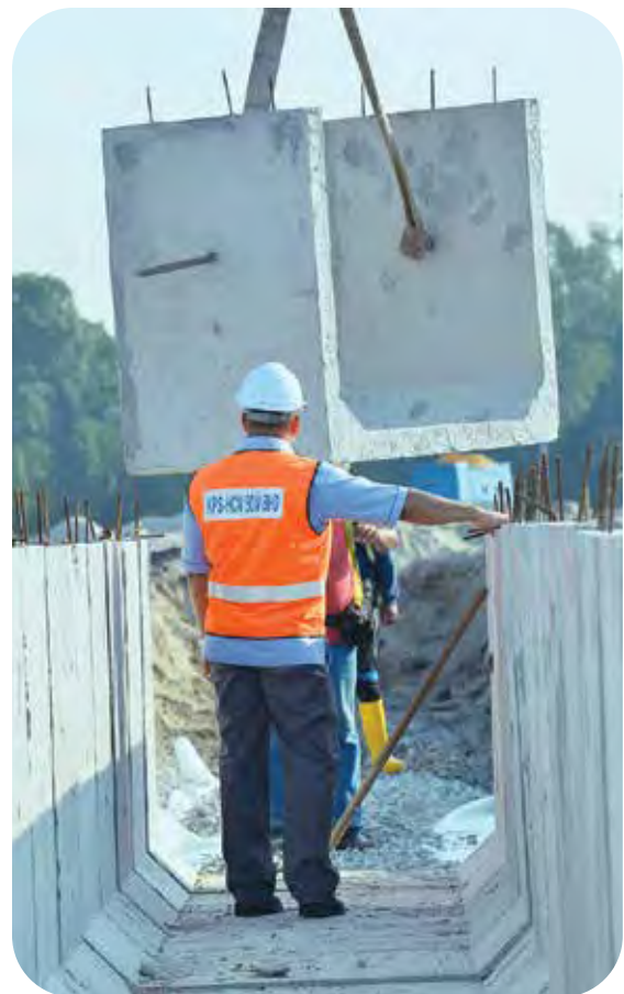
Drainage installation works at Phase 3C, Pulau Indah Industrial Park, Klang, Selangor.
