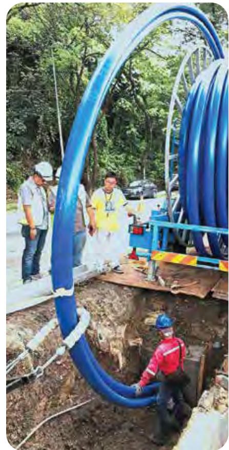
One of the Compact Pipe® installations for Pengurusan Air Selangor Sdn Bhd.
