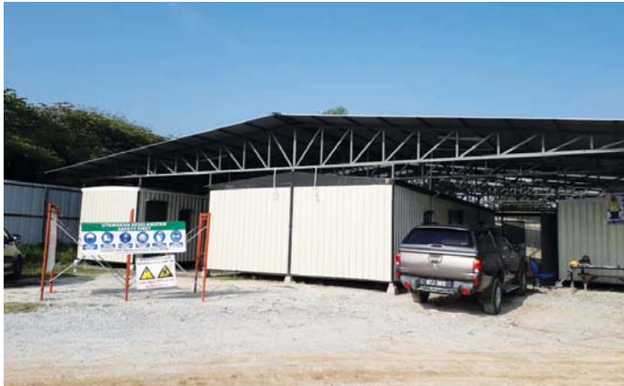
■ Setting up of site offices which comply to safety & health regulations
