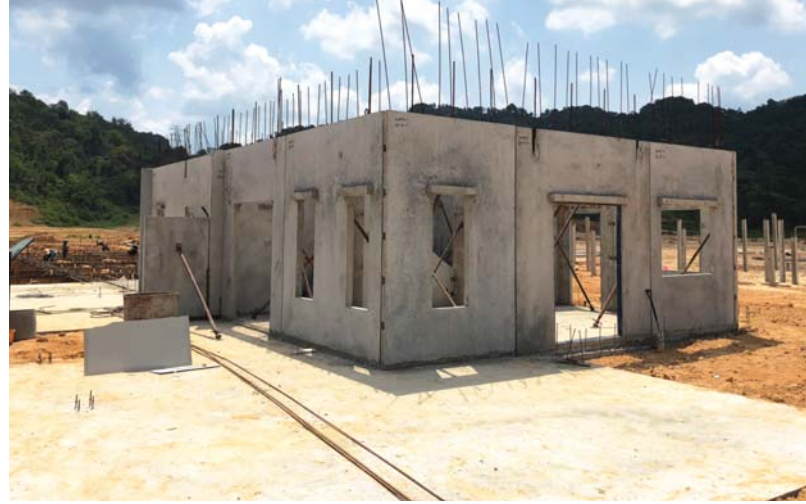
■ Construction of affordable homes using SEDCO Precast's product
