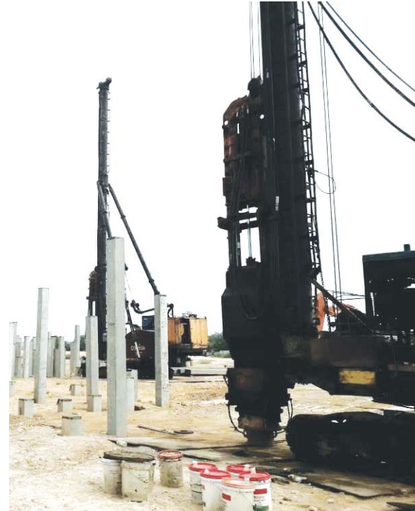
■ Drip plates below pile rig to prevent ground pollution.
