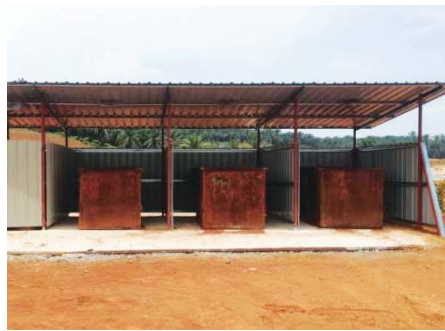
■ Recycling and waste segregation area at site office
