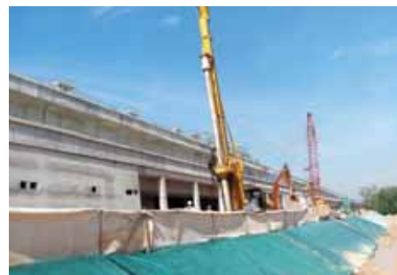
Slope protection and silt fence
