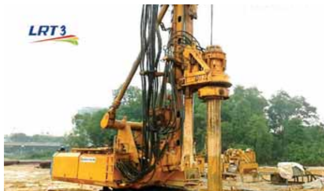
Bored piling works for LRT3 have commenced with project 4% completed.
