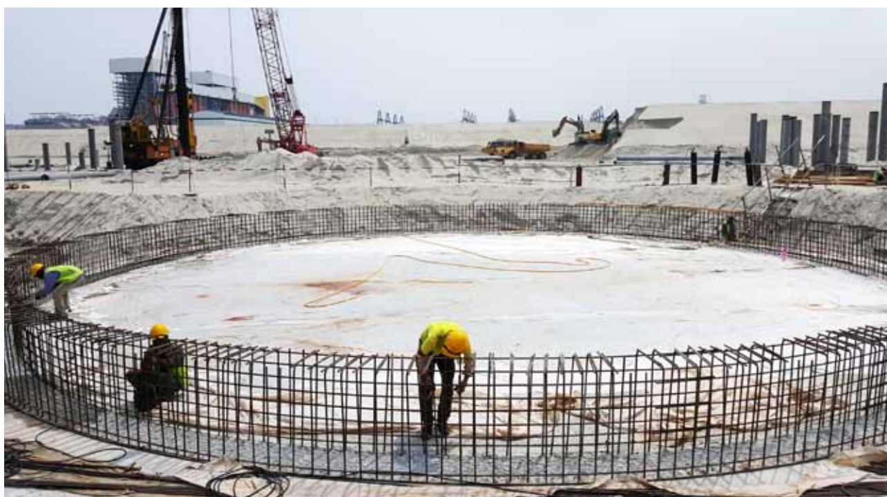
Water Tank Foundation at Jimah East Power (2x1000MW) Coal Fired Power Plant ("CFPP"), Port Dickson
