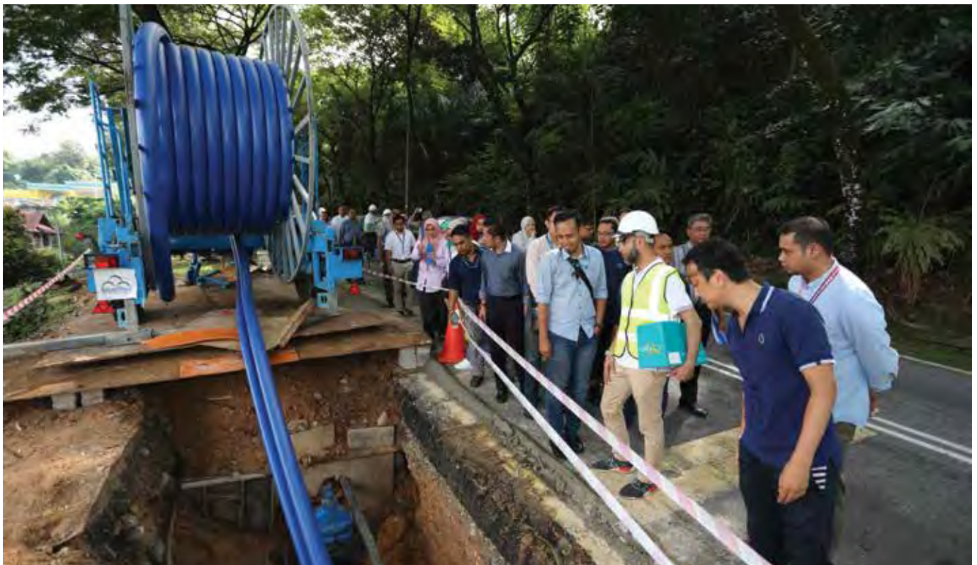
Smartpipe demonstrated the trenchless pipe installation system to Air Selangor officers at Taman Bukit Anggerik, Cheras, Kuala Lumpur.
