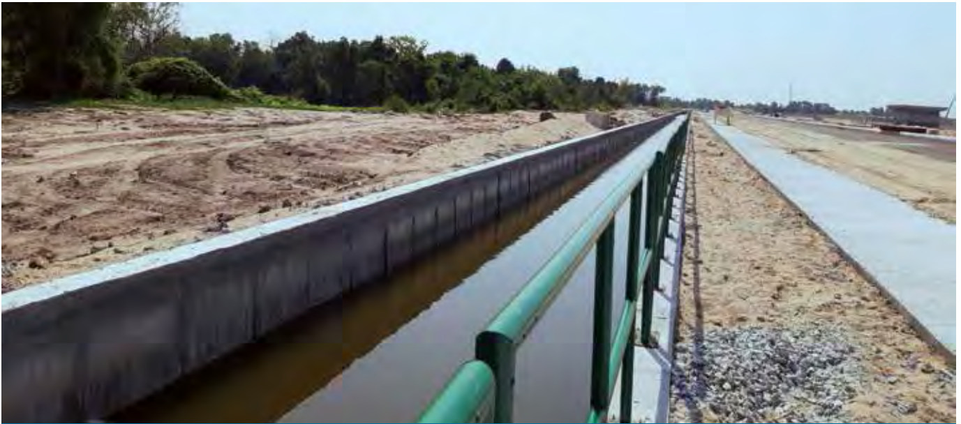
Installation of fiberglass-reinforced polymer railing at Phase 3C, Pulau Indah Industrial Park.
