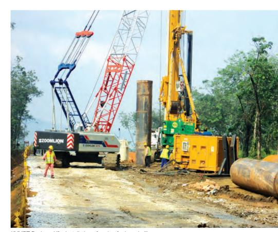
KVMRT Package V2 - Installation of casing for bored piling
