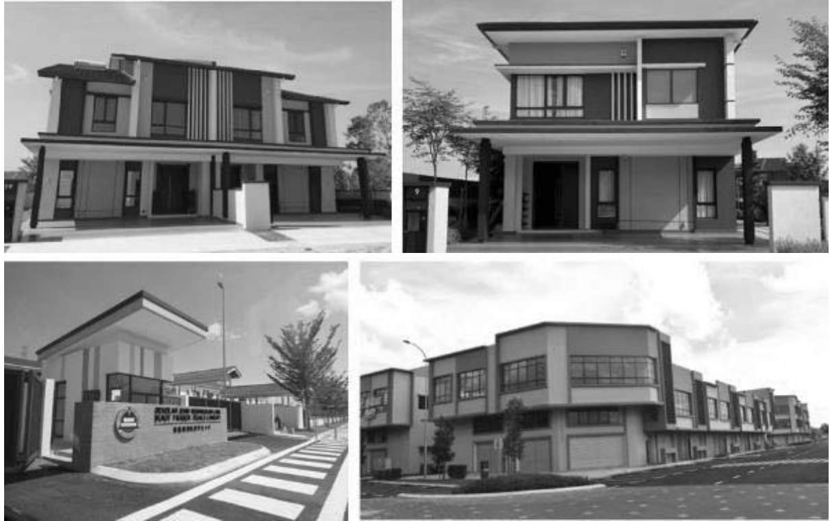
Top: Show houses (Tropicana Aman (Freesia Residences) Project); bottom left: School (SJK(C) Bukit Fraser); bottom right: 2-storey and 3-storey shop offices (Tropicana Aman (Triana) Project)
