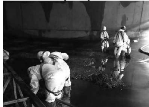
Cleaning storage tanks
