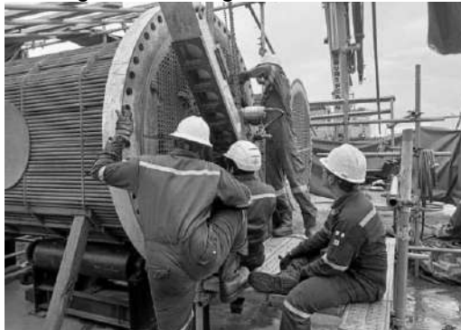
Cleaning heat exchanger tube bundles
