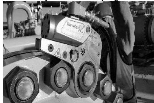
Hydraulic bolt torquing
