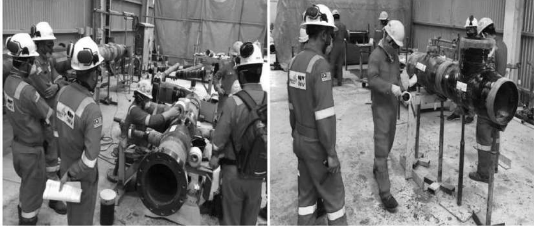
Fabrication of a pipe spool at our customer's facilities
