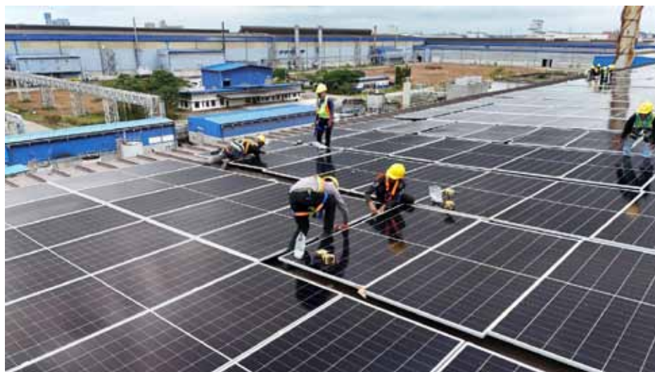
Installation of solar panels for one of our green projects
