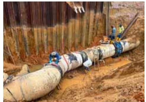
Rerouting existing water mains pipe
