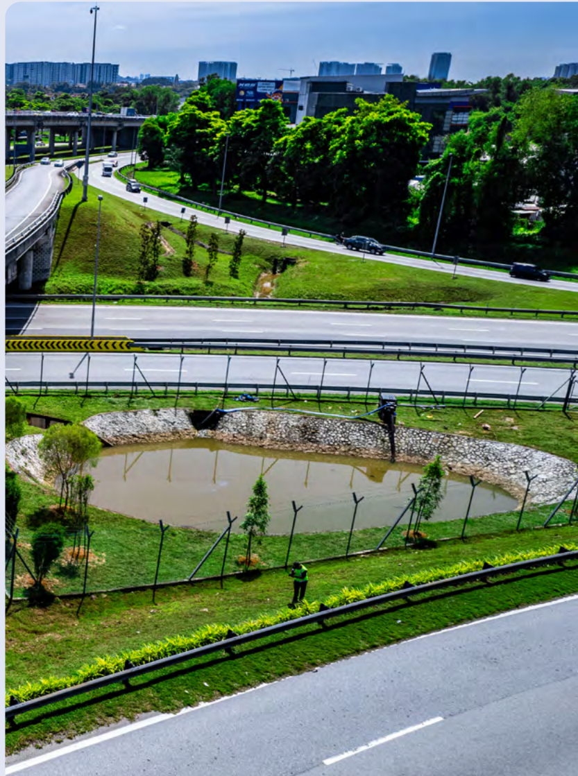
A retention pond along the GCE, supporting stormwater management, flood mitigation and a greener landscape.
