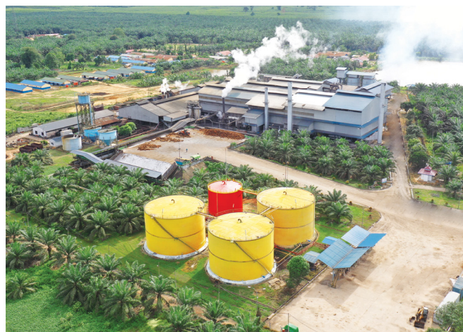
Aerial view of CPO mill and CPO and CPKO storage tanks
