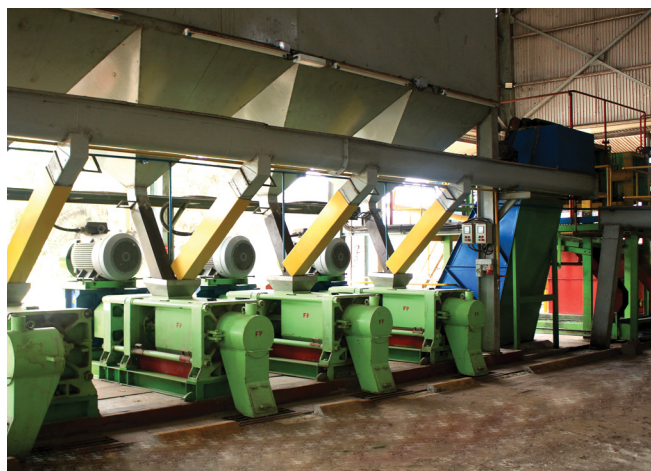
Palm kernel oil expeller installed at PK mill
