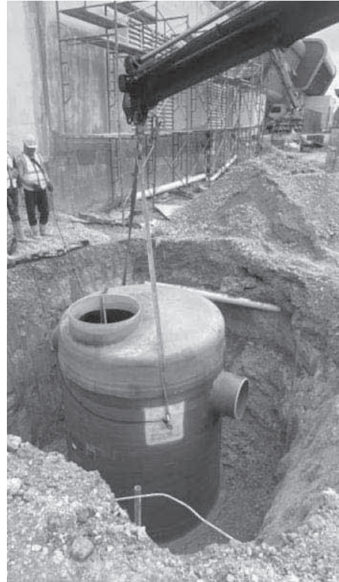
Installing an oil separator at one of our data centre projects
