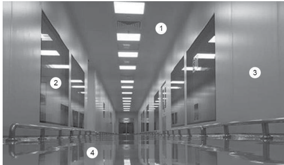
(1) Ceiling system with lighting and air return grilles (2) Windows (3) Wall partition system (4) Epoxy coated floor
