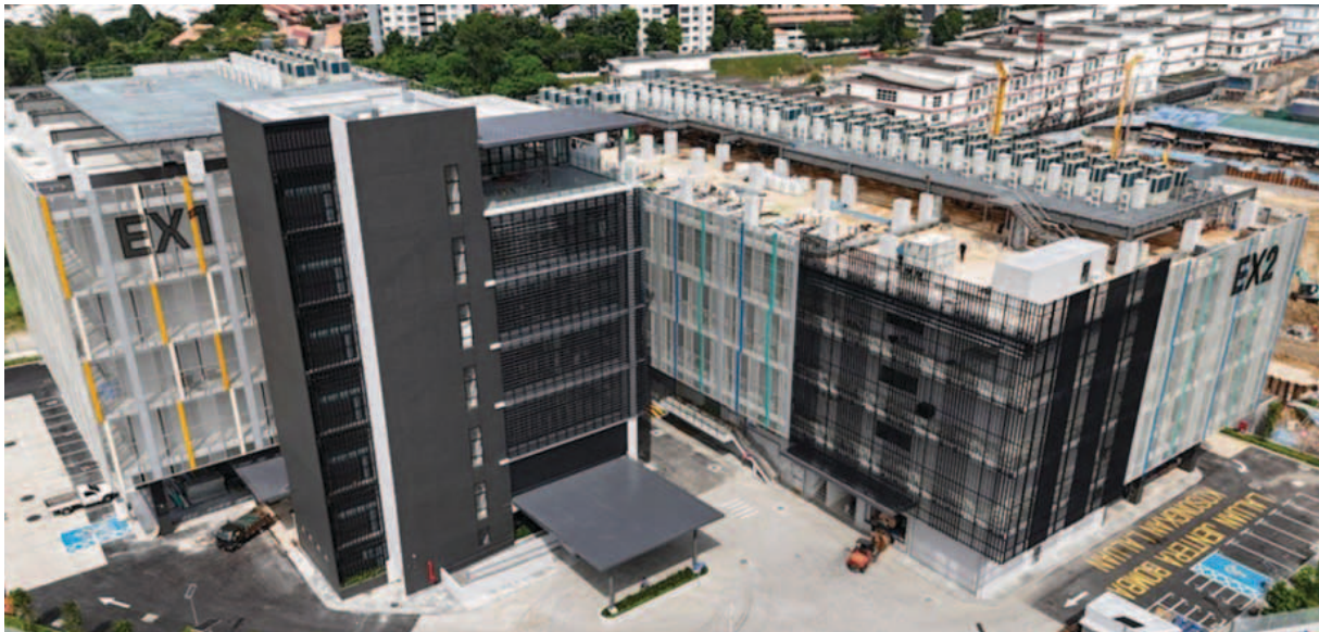
Exterior view of the completed façade of our first data centre project in Bukit Jalil
