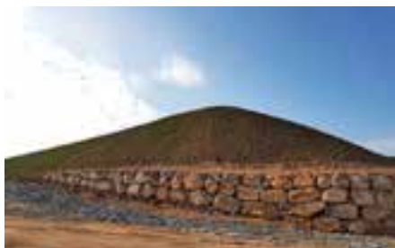
Boulders retention wall
