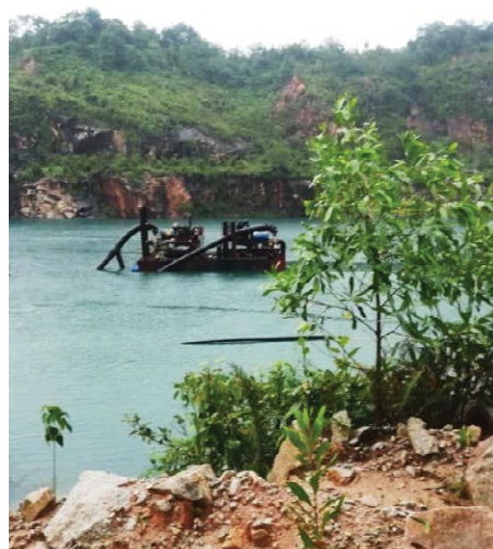
Raw water pumping system from Tasik Biru to Upper Layang Dam to increase the raw water storage volume
