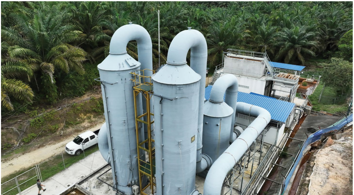
PRS System, Air Stripper and Gas Scrubber with Treatment Capacity up to 500ppm of ammoniacal nitrogen content
