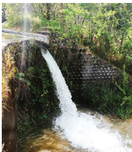
Outfall at Layang Dam from Tasik Biru raw water pumping system
