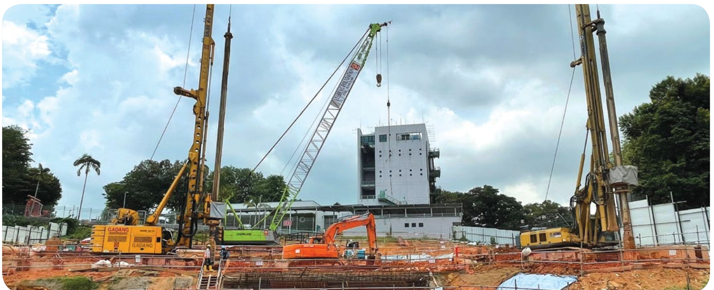
CAAS Changi: Foundation bored piling and secant bored piles work
