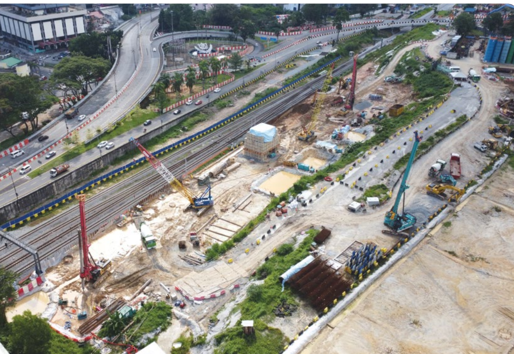
View of RTS Link Station Project – Bored piling works in progress
