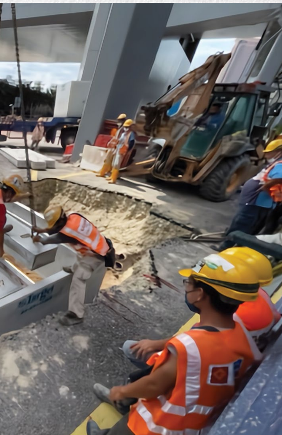
To supply and install modified TNB Manhole for TRX C3 project
