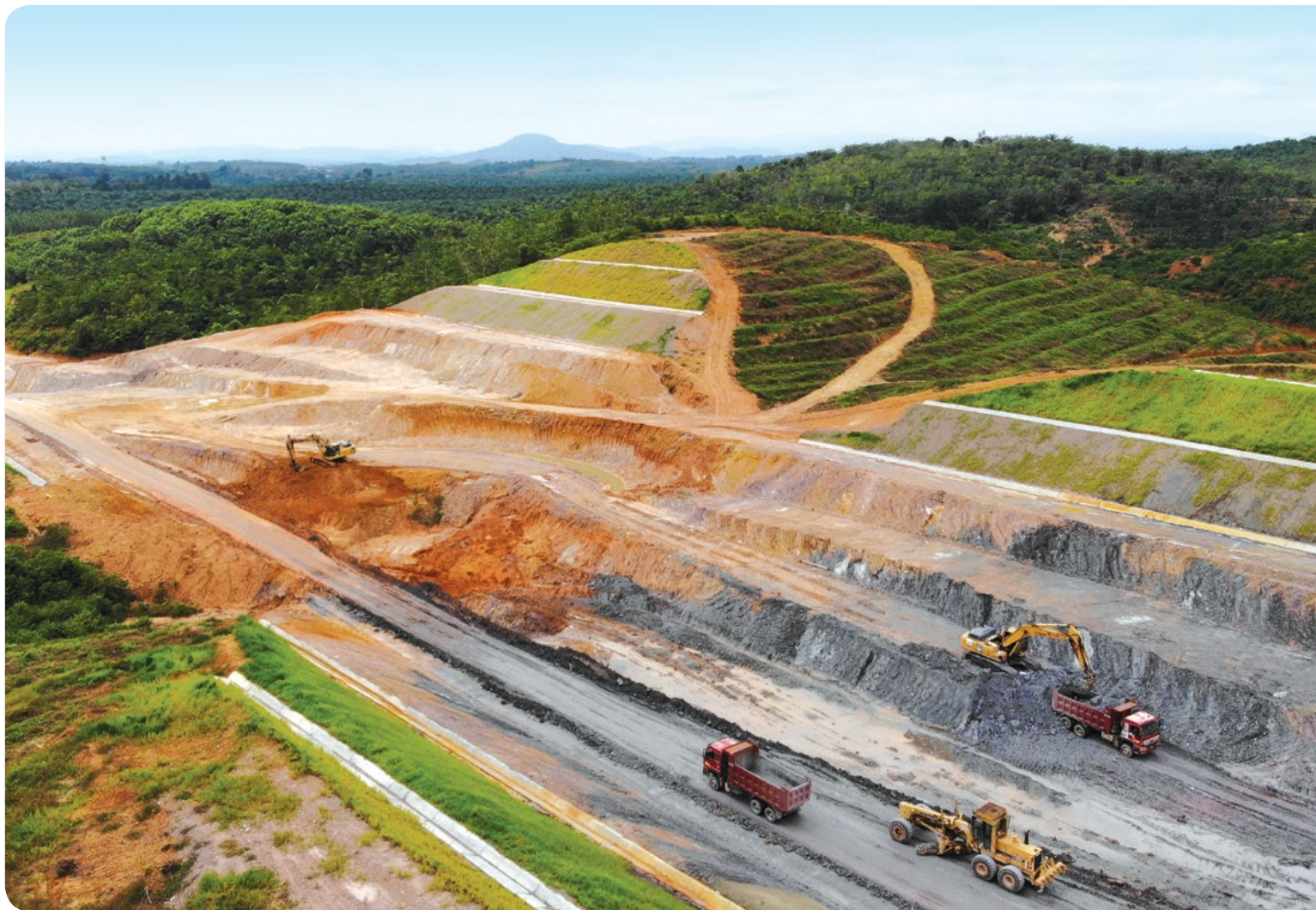
ECRL Section 6 (Maran - Temerloh): Slope cutting and forming the railway embankment
