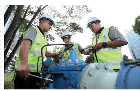
Ranhill field experts performing Pressure Management by adjusting pressure reducing valve
