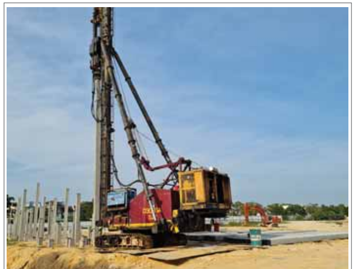
Drip plates below pile rig to prevent ground pollution at E'Island Lake Haven
