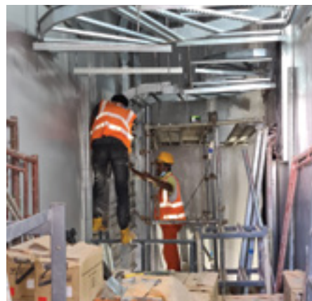
▲ Cable riser works in TRX tunnel
