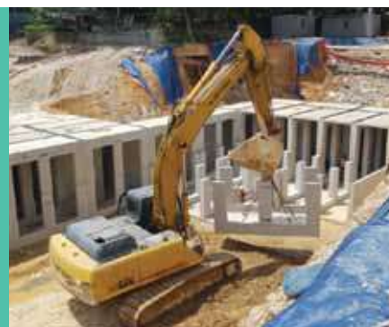
Picture: Lifting of G-Cast Eco-Modules (customised underground stormwater storage tanking system) for installation to On-Site Detention Project located at Taman Botani Kuala Lumpur own by DBKL.
