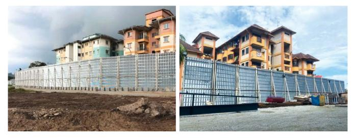
Silt traps are installed at the construction area to control total suspended solids and turbidity of water discharge from site into public drain. In-situ monitoring are carried out weekly and after rain event (rainfall more than 12.5mm) to ensure silt traps are working properly.
