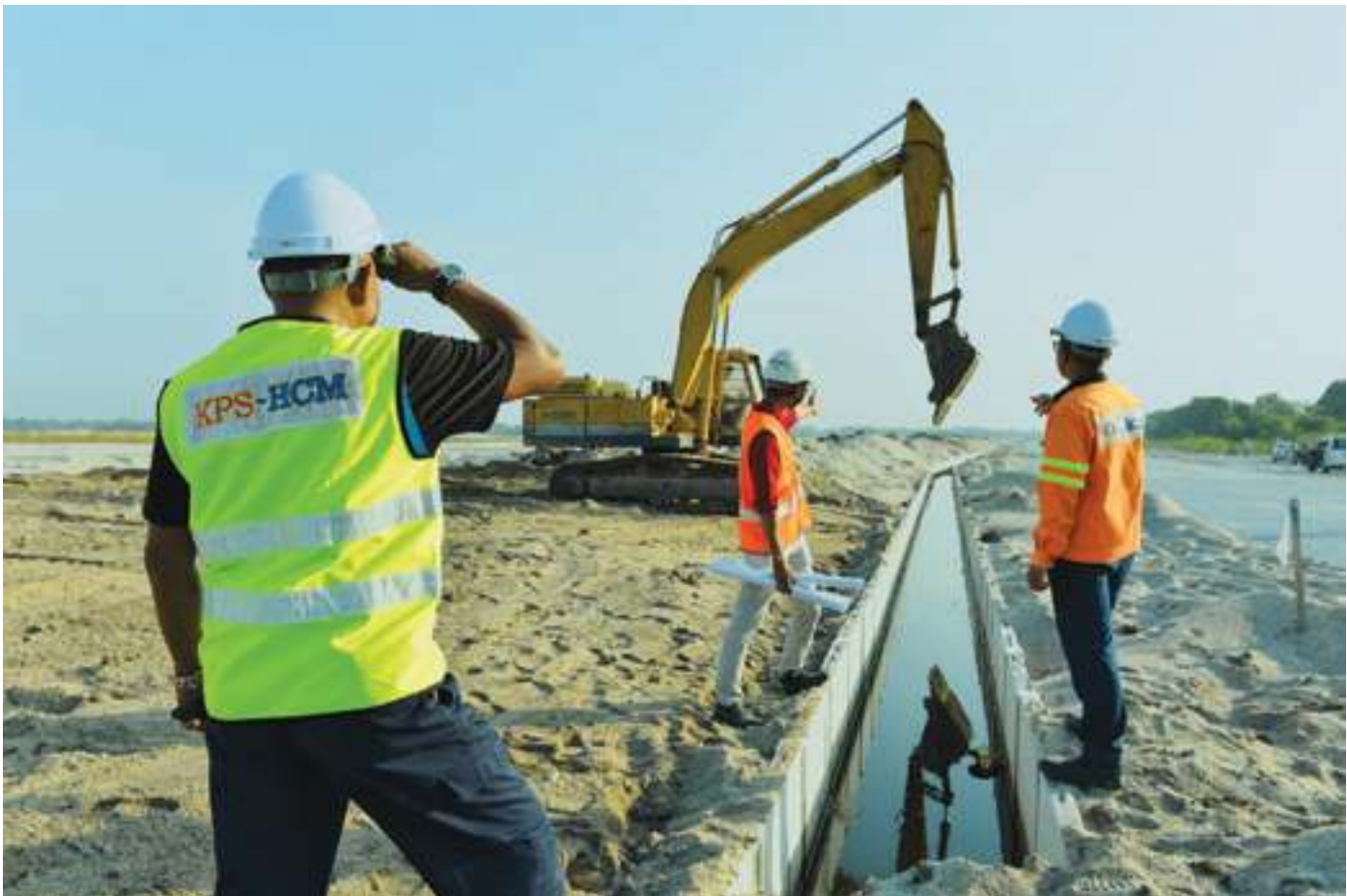
Drainage installation works at Phase 3C, Pulau Indah Industrial Park in Klang, Selangor.
