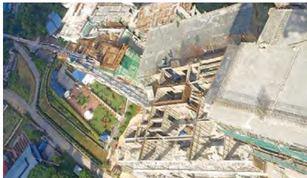
Aluminium Formworks at The Peak
