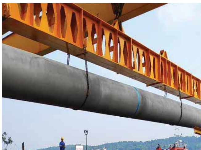
Loading of Marine Pile (1000mm x 48m single length) at Pasir Gudang Jetty, Johor
