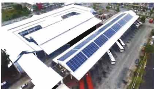
Rooftop - Retrofit installation
