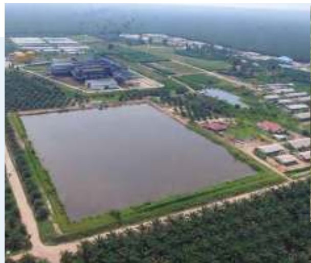
Mill effluents are treated in a designated area at the mill and recycled as natural soil fertiliser
