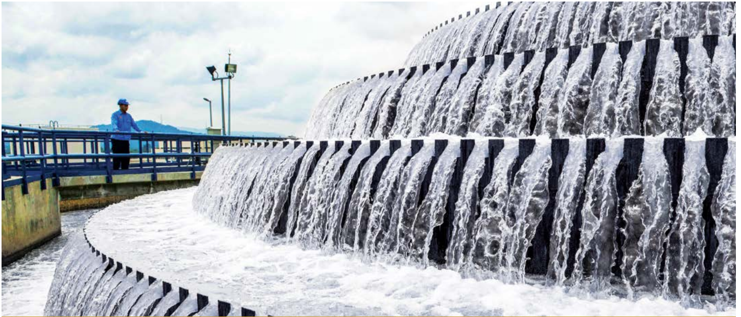
Aerator in Semanggar Water Treatment Plant
