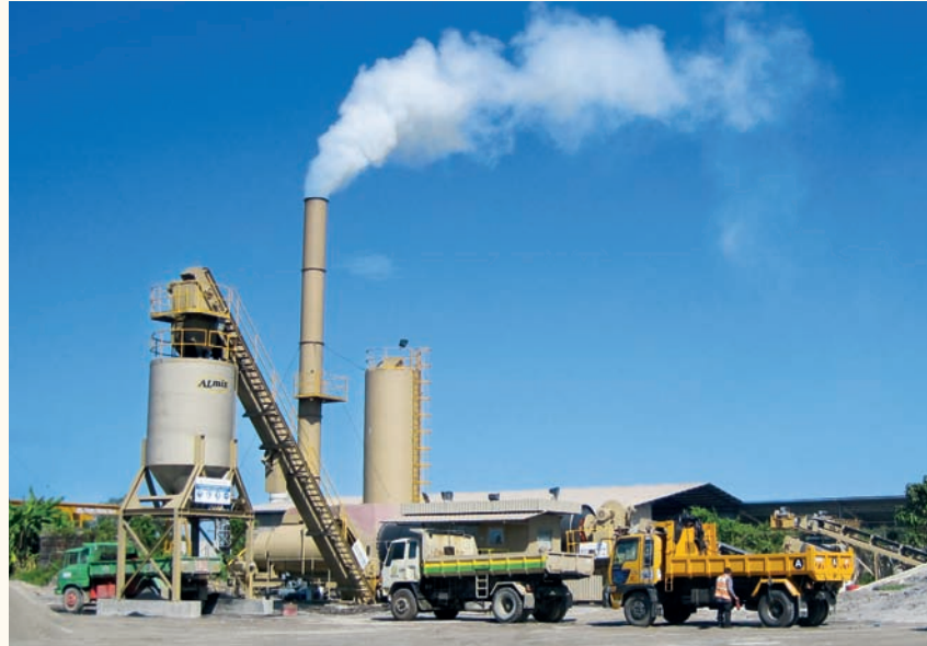
CMS Premix (Miri)'s new RM2.5 million plant comprising kiln, chimney, air filter, 40-tonne silo and tanks. Located at the company's premises at Lambir on the outskirts of Miri, the plant has a production capacity of 150 tonnes per hour.
