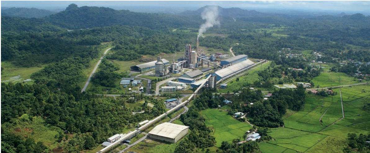
The CMS Clinker plant at Mambong, located approximately 21 kilometres from Kuching. The plant occupies 24.8 hectares of industrial land and has another 78 hectares of neighbouring quarry concessions.
