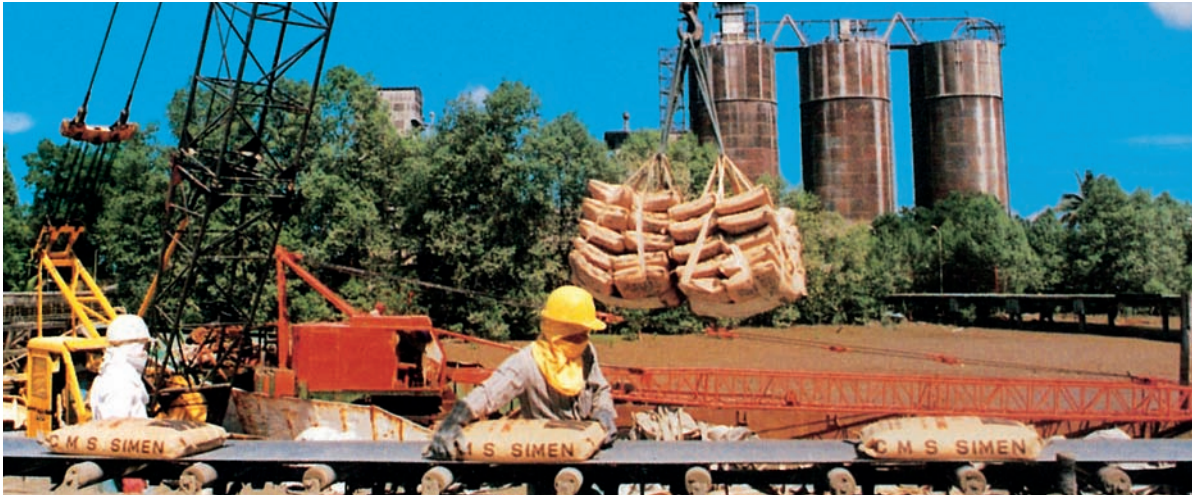
Loading 50 kg bagged cement at the Pending plant, 1994.
