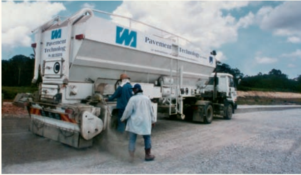
CMS's newly acquired prime mover and Australian-manufactured cement spreader deposits cement for in situ cement stabilisation.
