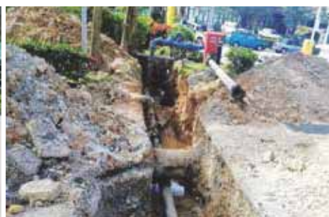
Figure 30: Replacement of underground domestic piping
