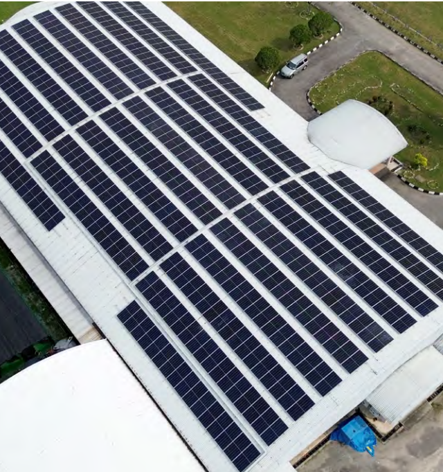
» Rooftop solar PV system under Net Energy Metering (NEM) scheme with Power Generation of 342,669 kWh/year installed at SD Guthrie's R&D centre at Banting, Selangor, Malaysia.
