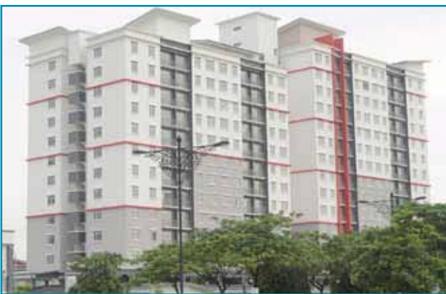
PR1MA project at Precint 11, Putrajaya
