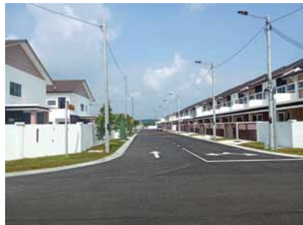
Newly completed Amber Phase 3 was handed over with vacant possession in March 2026
