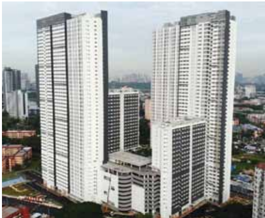
Newly completed 2 blocks of 1,192 units of apartments at Bandar Tun Razak, Kuala Lumpur
