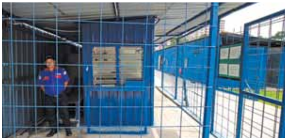
Guard house with 24 hours security
