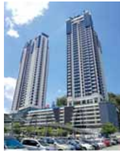
Wangsa 9 Residency - phase 1 completed in March 2019
