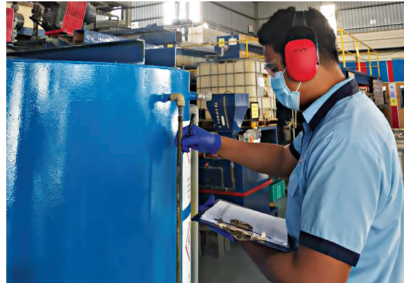
Environmental competent person performing checks at wastewater treatment plant
