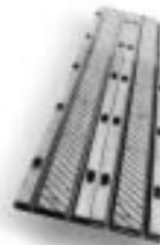
• Bridge Expansion Joint
