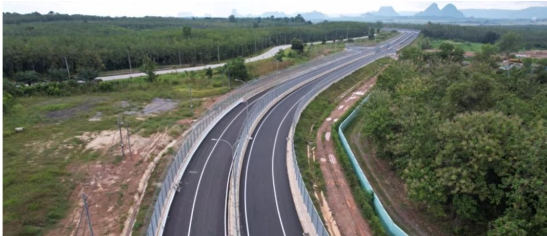
Figure 3: Completed Bonded Road
