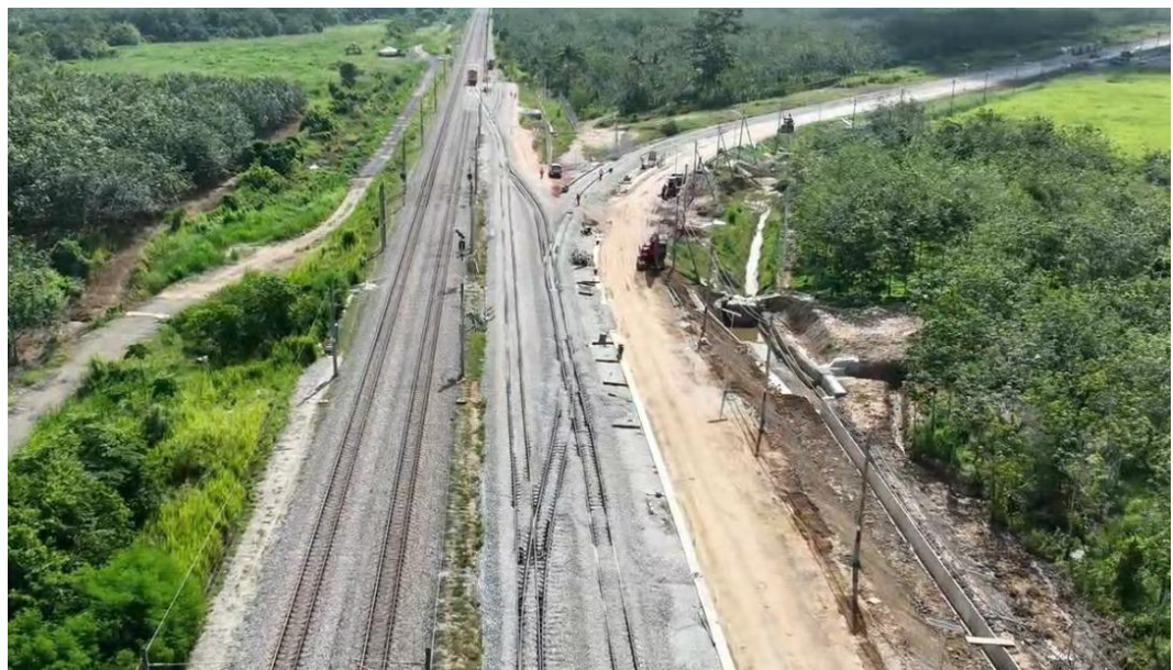
Figure 4: Completed Spur Line
