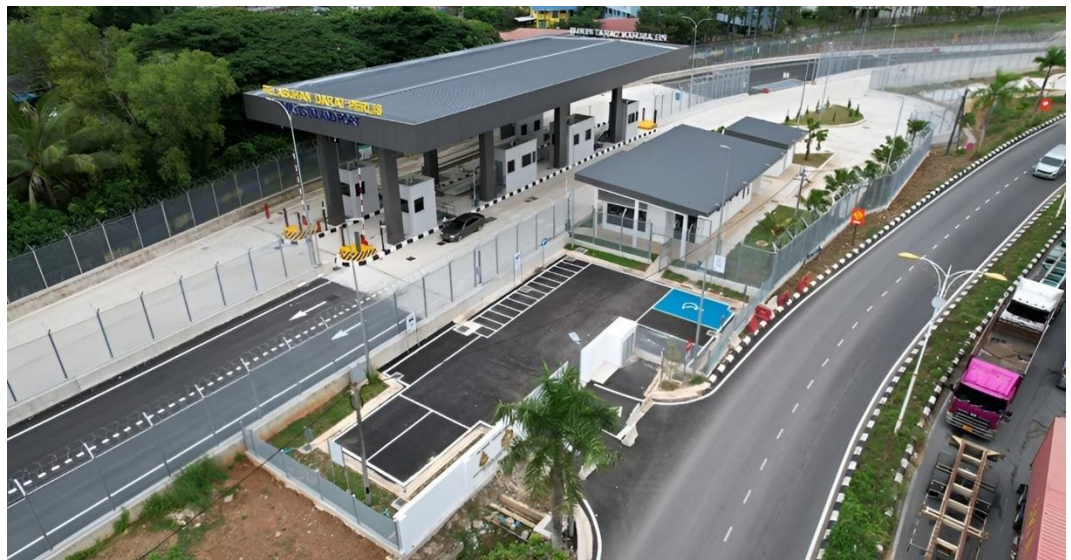
Figure 2: Completed Checkpoint at PIP
