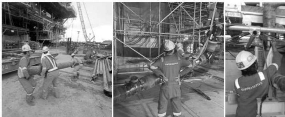
Installation of pipe spool on the offshore platform at our customers' fabrication yard in Pasir Gudang, Johor
