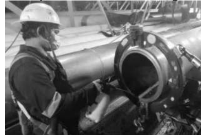
Pipe cold cut and bevelling
